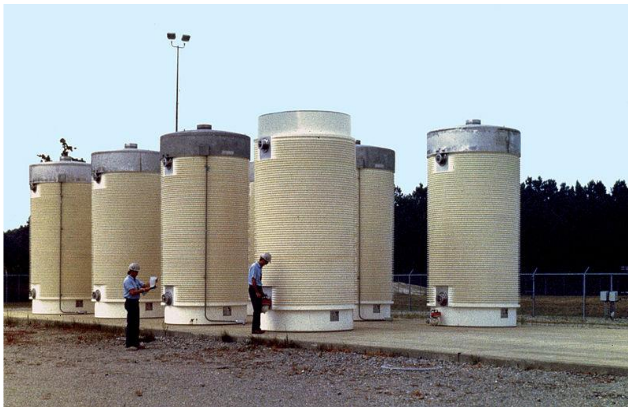
Figure 14. German Dry Casks are Used for Spent Fuel after Five Years in a Pool Germans have been using Dry Casks for 15 years. File from Wikimedia Commons.
