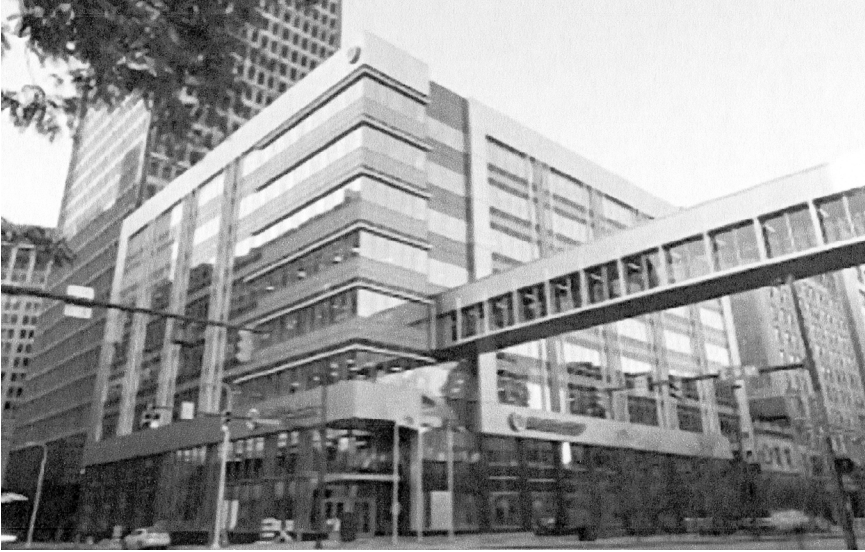
County Administration Building
