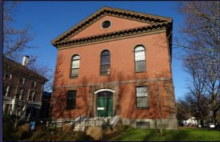
Town House Exterior Restoration and Accessible Entrance (2006, 2009, 2012, 2013)
