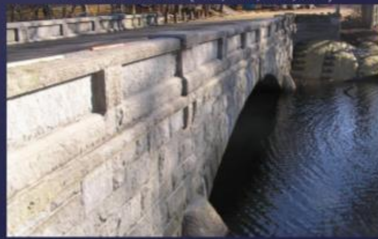
Nashawtuc Bridge Restoration, Town of Concord (2008)
