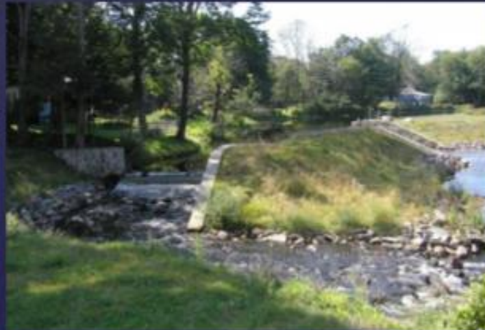
Warner's Pond Dam Town of Concord (2006)
