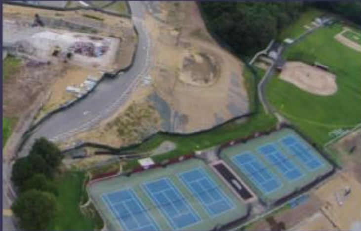
CCHS Field Renovations, Phases I, II, III CC @ Play (2014, 2015, 2016)
