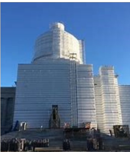
Watch for construction on Missouri's Capitol building.
