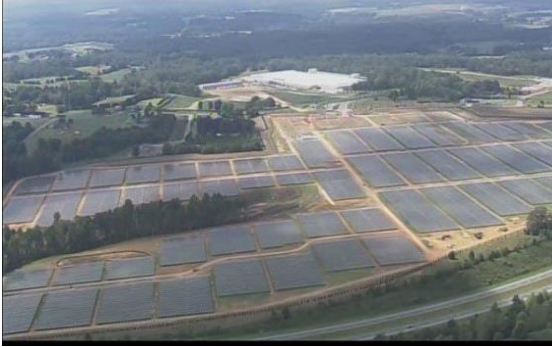
Pictured: California Flats Solar Project, Monterey County, California
