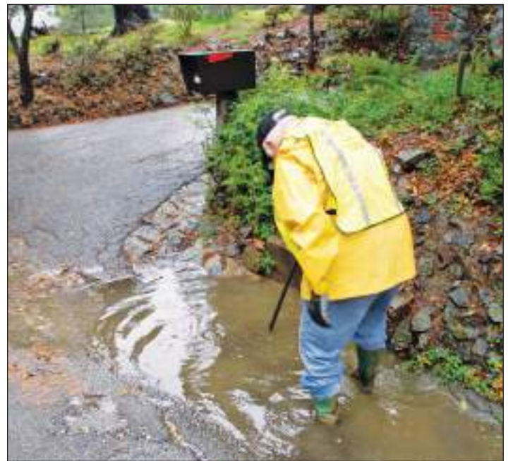
Adopt a Drain volunteer Peter Crigger unclogs a storm drain in his Oakland neighborhood.
