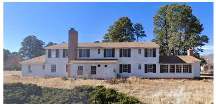
Women’s Dorm Building east elevation facing 17th Street, Google Earth Street Image, November 2022
