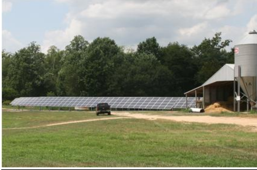
Figure 2. Roof mounted and ground mounted residential and commercial PV systems in Delaware. The residential homes are 6.2 kW and 1.8 kW (upper left and right, respectively); the church is Limestone Presbyterian (18 kW). The ground mount is 2.4 kW, all in New Castle County. The bottom photo is a poultry farm (63 kW) in Ellendale in Sussex County.
