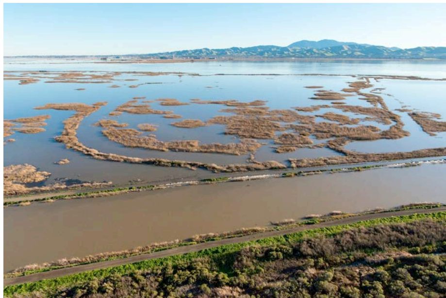
Roaring River levees overtop at Grizzly Island in Solano County, in the Sacramento-San Joaquin Delta, January 13, 2017. (Florence Low/California Department of Water Resources)
